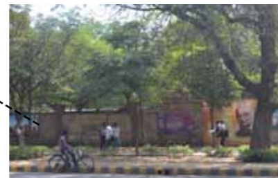
Boundary Wall, Doordarshan Bhawan, Copernicus Marg
