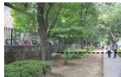
Boundary Wall, Ravindra Bhawan, Copernicus Marg
