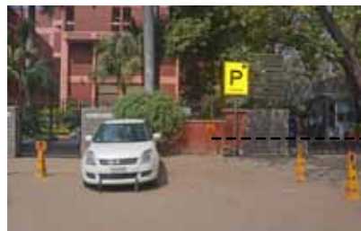
Boundary Wall, Shri Ram Bhartiya Kala Kendra, Copernicus Marg
