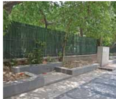
Pedestrian walkway, Police Headquarters, New Delhi
