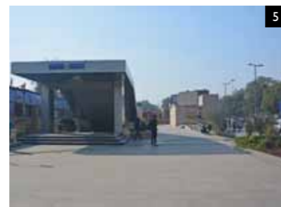
Metro Entry/ Exit
